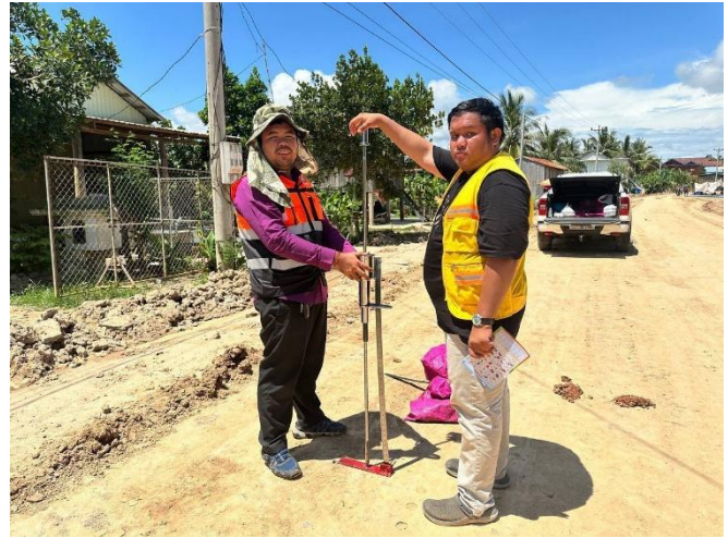
Fig. 2. Dynamic Cone Penetrometer (DCP) testing at the site
